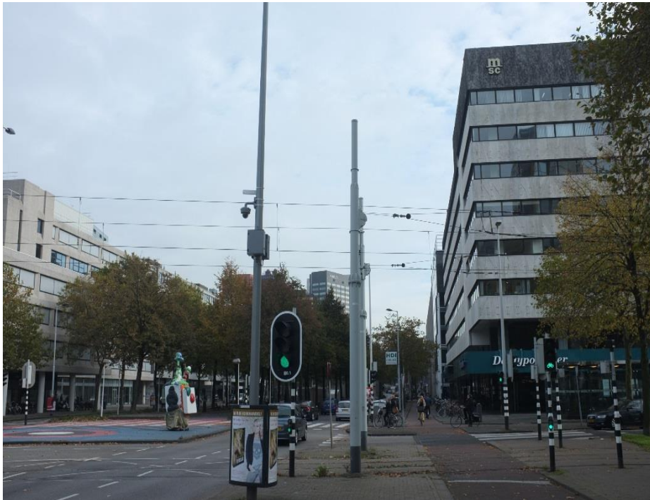
Figure 26: 'De Eendracht' office building (the building on the right in the picture): control tower of the port of Rotterdam
