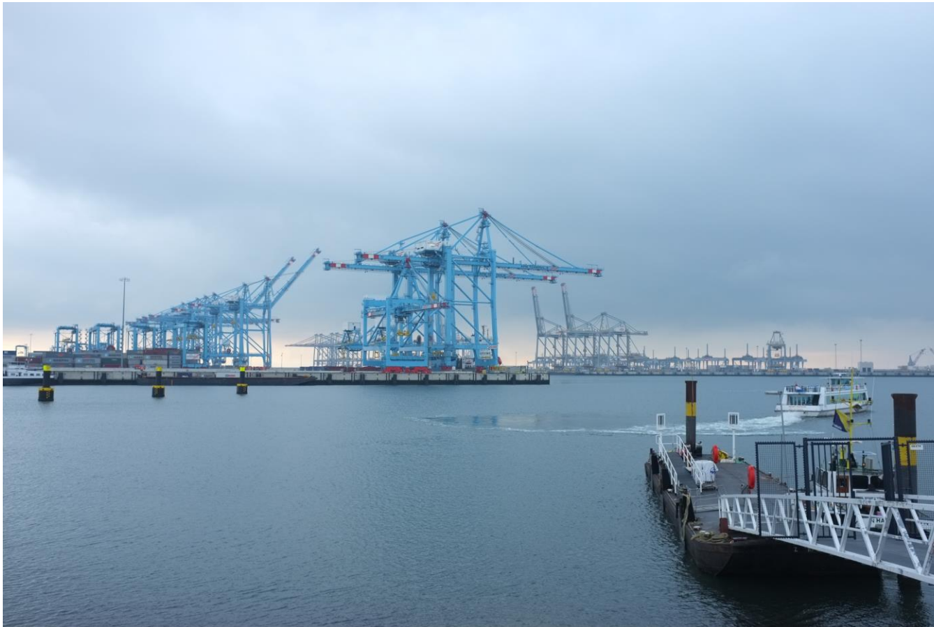
Figure 3: APM Terminals Maasvlakte 2 terminal is based on wind-power generated electricity. The new 2.7 million TEU annual capacity deep-sea facility is claimed to be the world's first terminal to eliminate container handling equipment emissions: an electric-powered personnel vehicle fleet and terminal electricity will be 100% sustainably-sourced.
