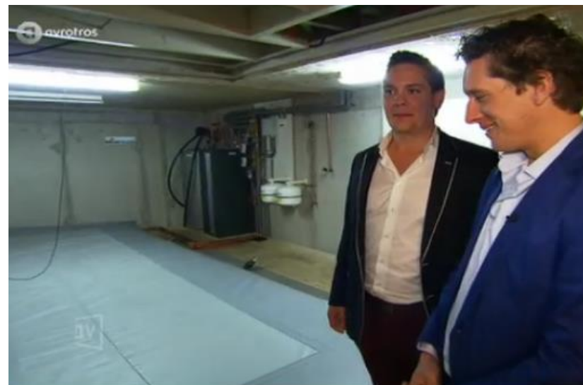
Figure 6: Solar Freezer: 'waterbed' stores solar energy. Source: https://www.youtube.com/watch?v=oPWemUa8ots
