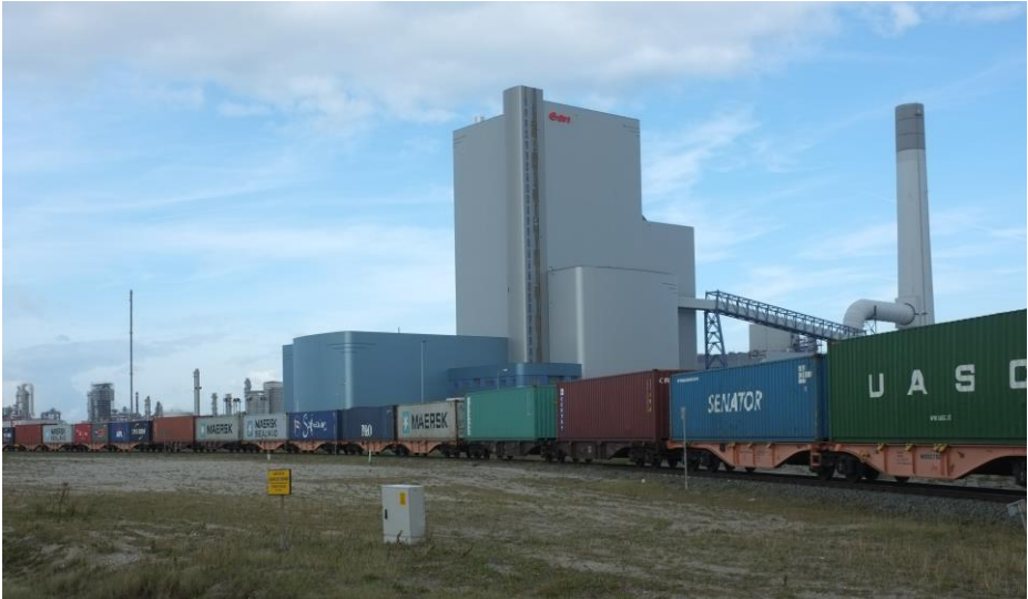
Figure 4: In 2015 two new coal-fueled power plants started their operations in the port of Rotterdam (Eon and GDF Suez). The decision-making behind the construction is a very obscure process including issues like energy-independence and privatization of electricity markets in the Netherlands. However, these new power plants are part of the national ‘energy deal’ in the Netherlands and replace some older and less efficient coal fueled power plants.
