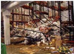
Forklift Collision with Storage Racks
